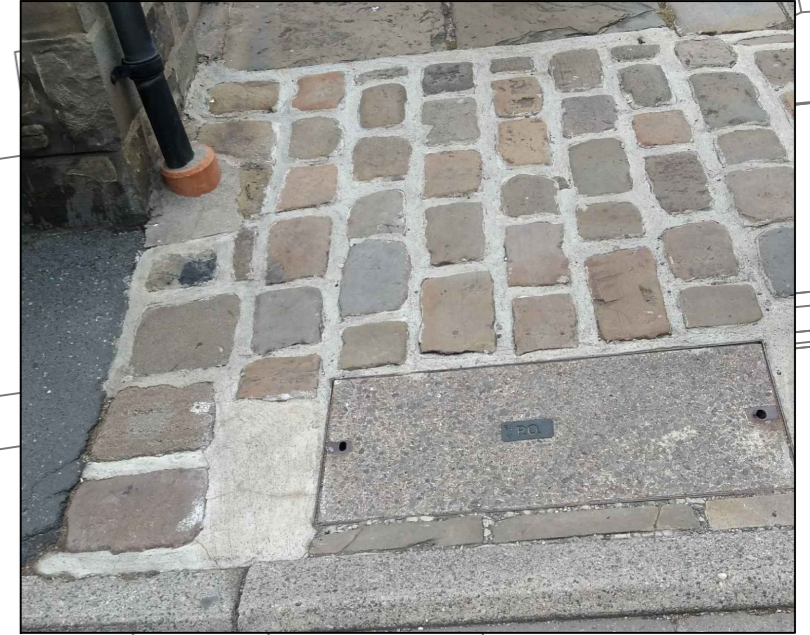
HISTORIC SETTS TO BE CLEANED AND RE-POINTED CONCRETE SERVICE COVERS REPLACED WITH STONE INSET COVERS
