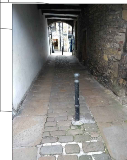
DE-CLUTTER GINNEL NEW SIGN AND LIGHTING
