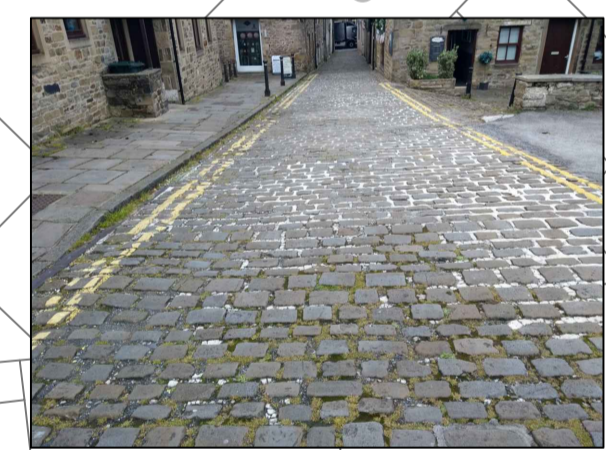
RESET STONE SETTS AND PROVIDE FLAGSTONE CENTRAL WALKWAY
