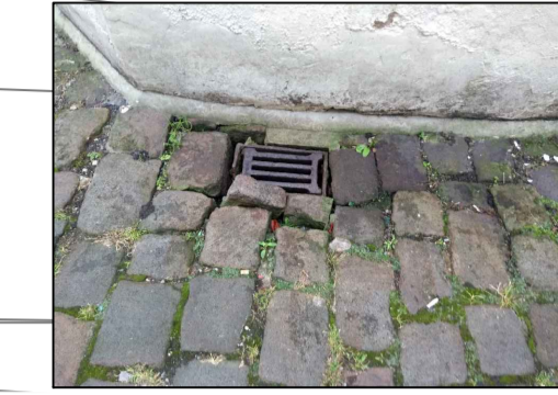
REVAMP YARD DRAINS, NEW PAVING SLABS, RE-SET SETTS
