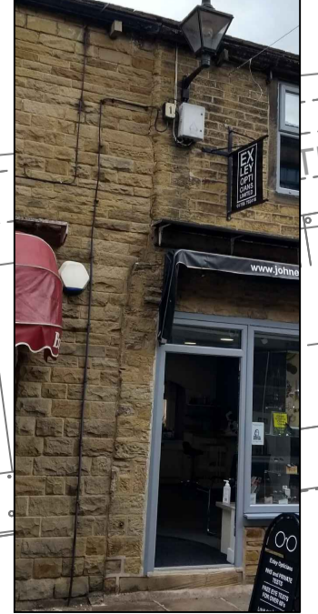
HERITAGE STYLE WALL MOUNTED LIGHTING UNIT ON OTLEY STREET
