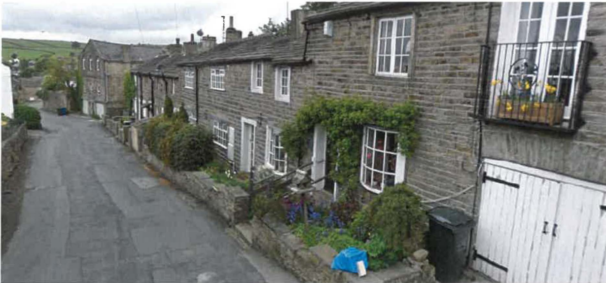
Figure 18: Crag Lane, casement windows on the upper levels
