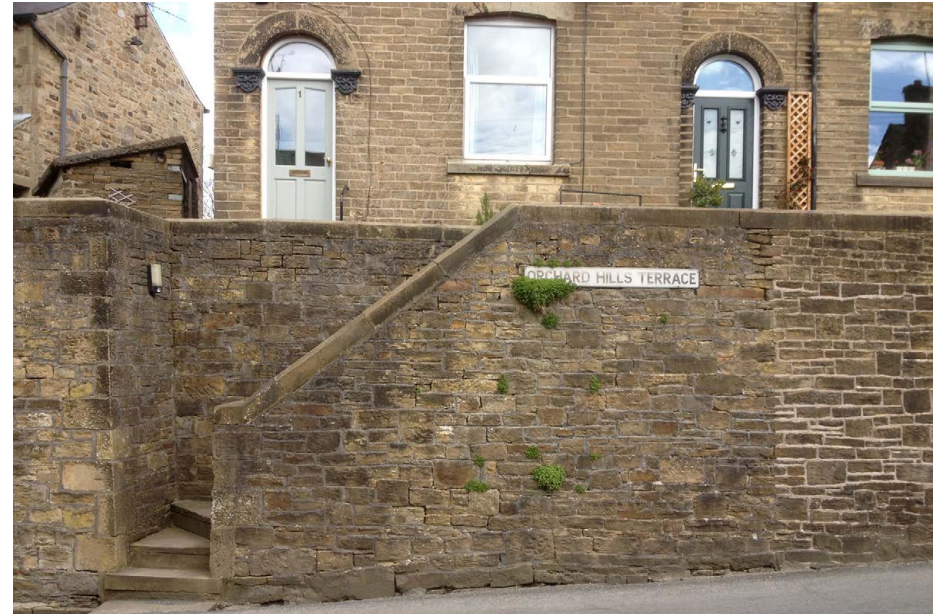
Orchard Hills Terrace. Note the separation from the road
