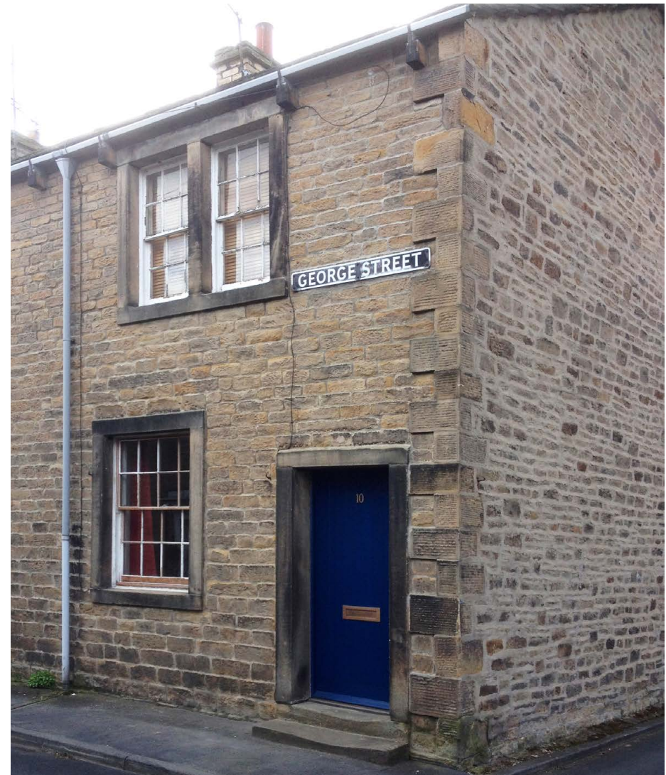
Surviving and cared for historic timber sash windows and traditional timber door on George Street
