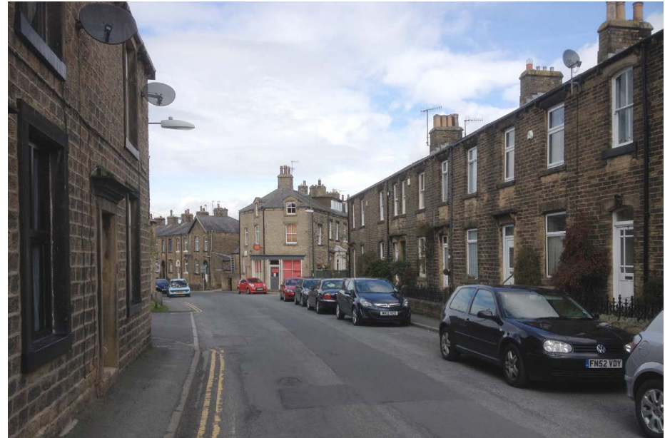
Late 19th century terraced housing on Swan Street
