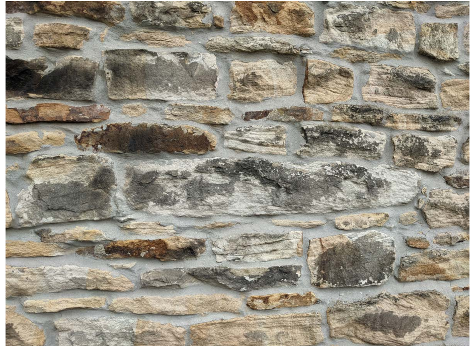
An example of coursed gritstone rubble construction in Cononley
