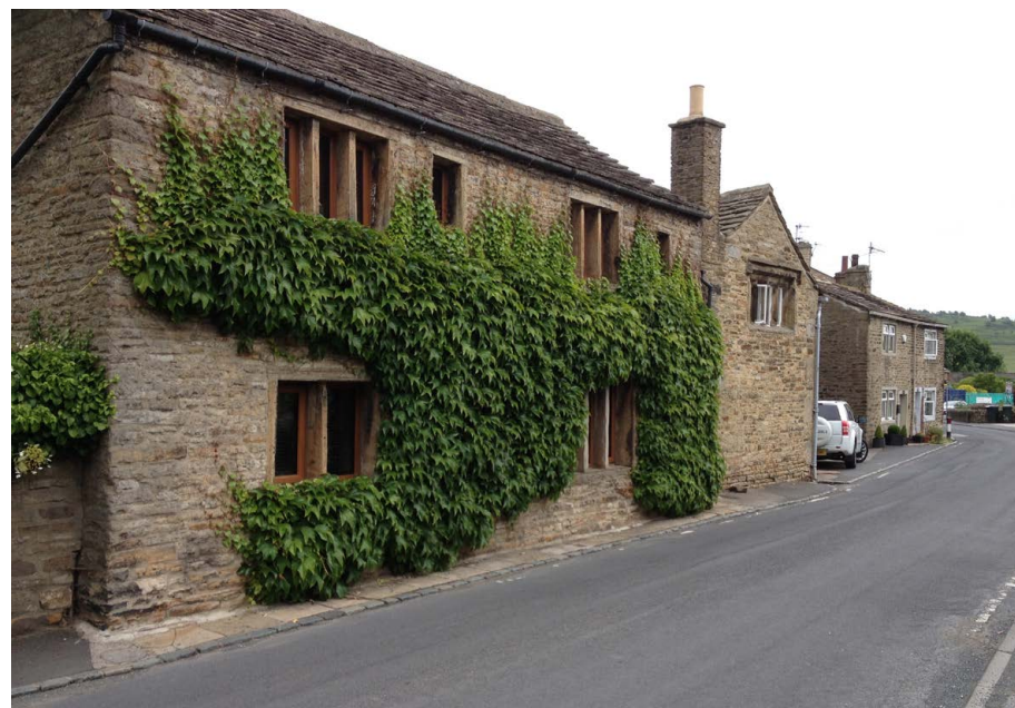
Sensitive restoration on Main Street
