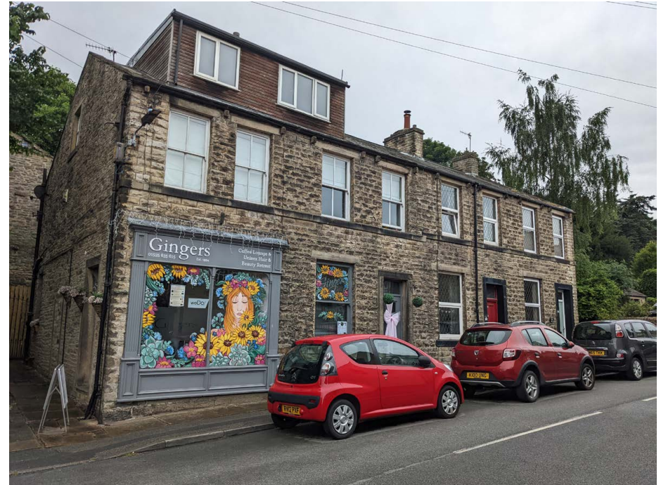
On the Main Street. Note the large dormer, timber sashes and upvc windows
