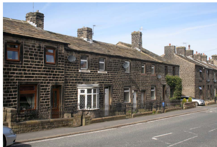
Typical historic terrace on Keighley Road with a variety of replacement windows
