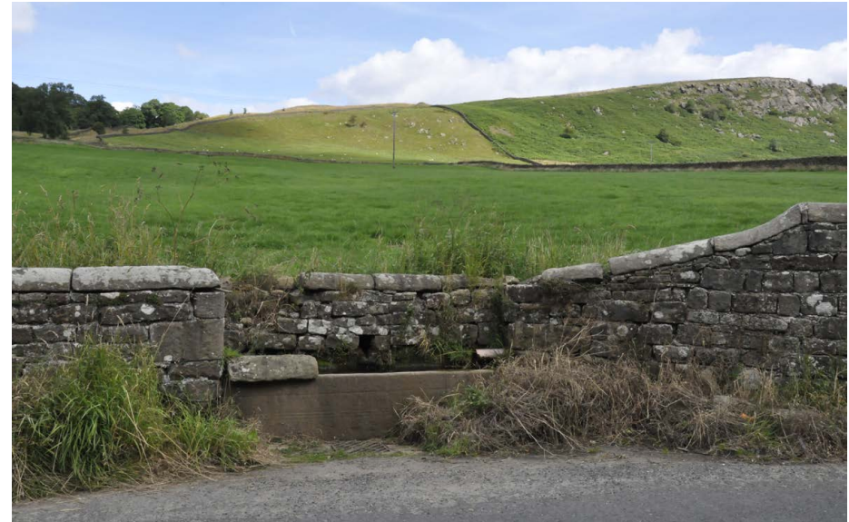
View into the National Park to the north of Barden Road showing a surviving historic water trough built into the field wall
