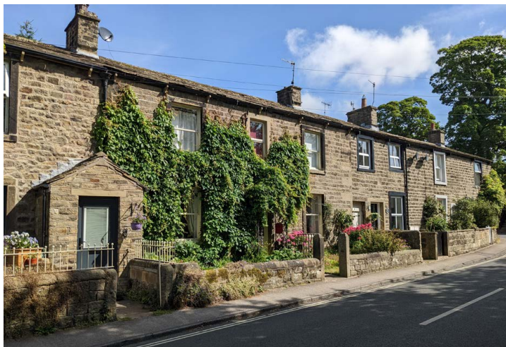
Row of cottages on High Street with a mix of upvc and timber sash windows
