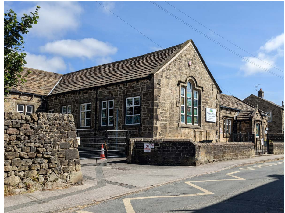
Landmark primary school on Pasture Road
