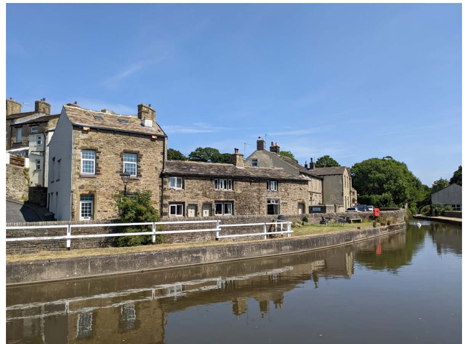
The grade II listed 15, 16 & 19 Newby Road with the canal in the foreground
