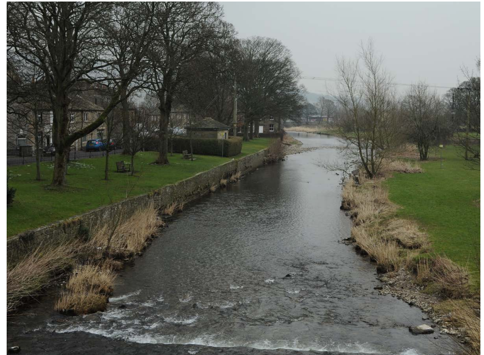
V1 - View of the River Aire looking east from the bridge in winter
