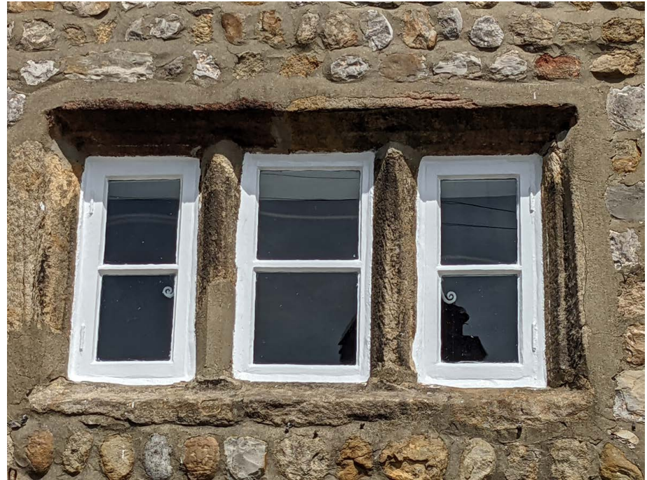
The same terrace on North Street with a timber casement window
