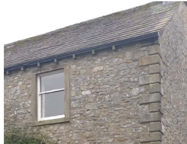
An example of the use of millstone grit in historic building construction
