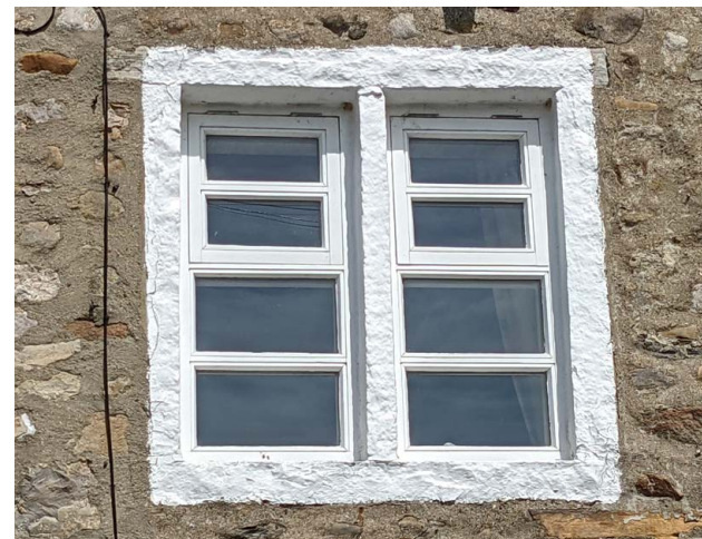
UPVC replacement window in a terrace on North Street
