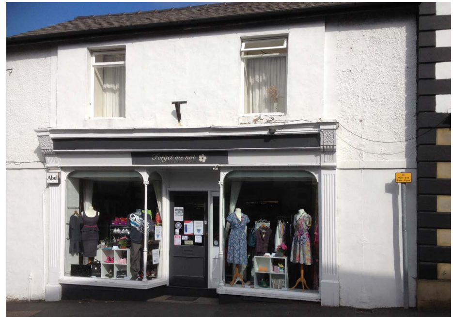
Historic shop front with first floor timber casement windows replacing historic timber sashes
