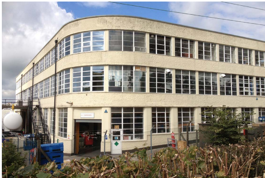
The 1920's Kidde factory building
