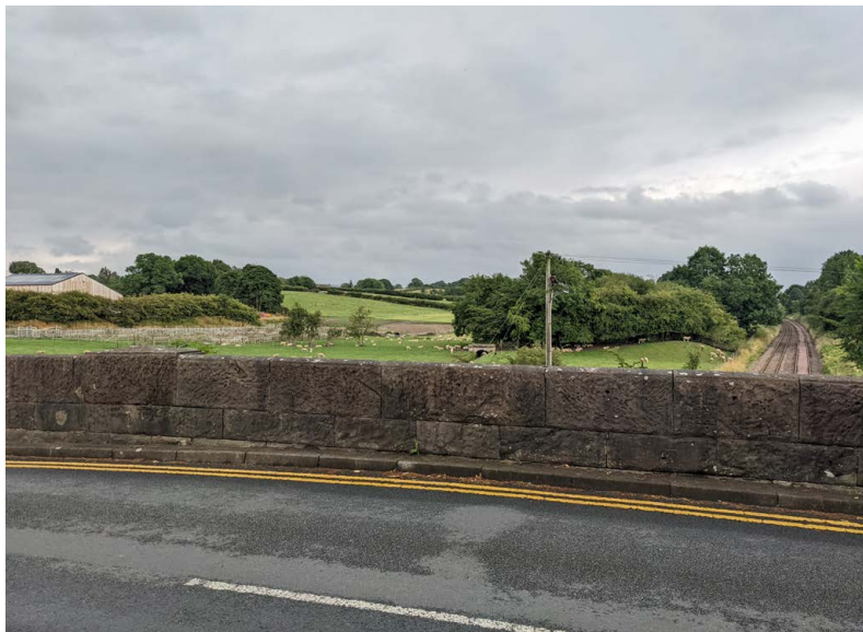
A view of OP3 from the Railway Bridge on Station Road
