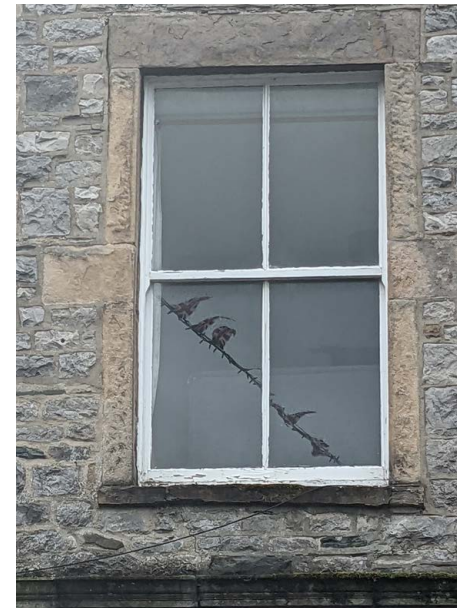
Detail of an historic timber sash window in Ingleton
