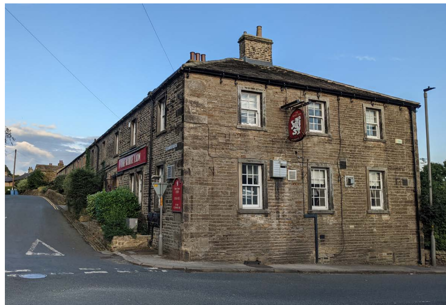
The White Lion public house in September 2021. Note this is closed but is now open (July 2022). Also note the view up priest Bank Road from its junction with Main Road
