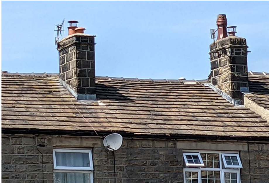
Strap pointing, stone tiles and upvc windows on an historic property in Kildwick
