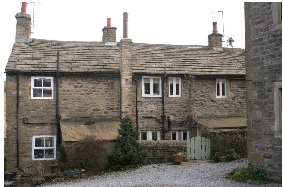
Replacement windows on an historic property in Wedding Hall Fold. Note the original stone tiled roof
