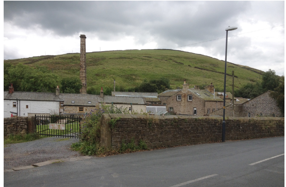
V10 – a view of the Dale End Mill from Rook Street
