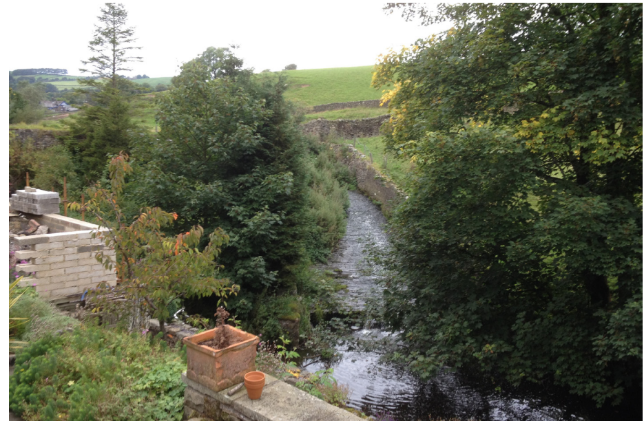
V9 – a view of the Dale End Mill water management system from Rook Street
