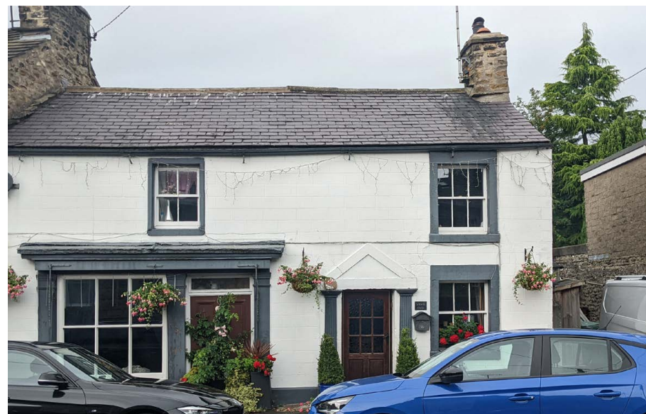
The grade II listed, "The Old Post Office". Note the restored and conserved traditional timber sashes and shop front
