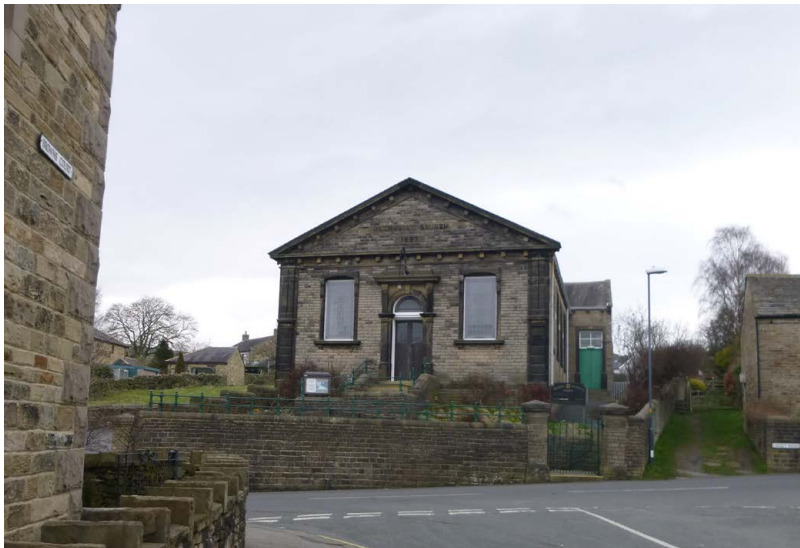
Methodist Church, Skipton Road
