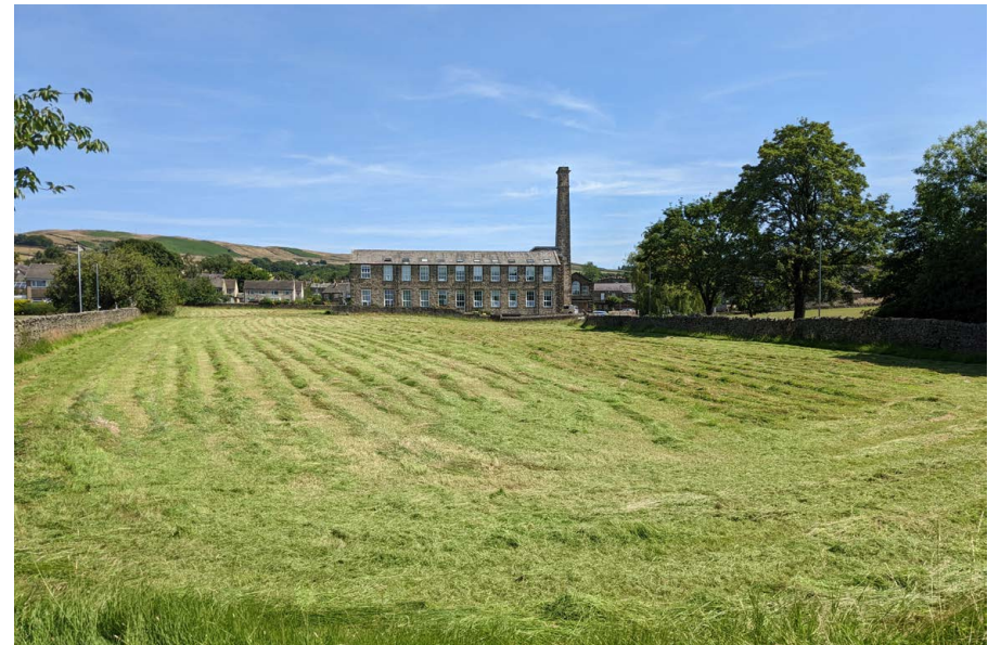
V1 showing Bradley Mill and its open context (OP9) from Ings Lane
