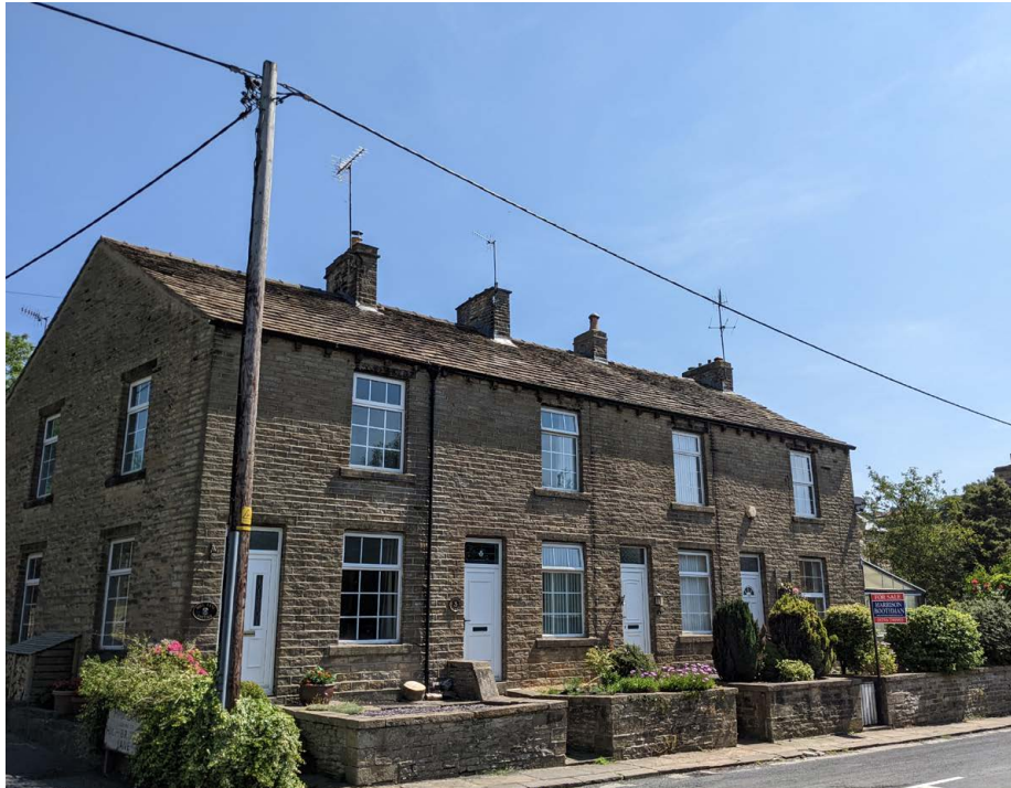
A typical example of replacement upvc windows and doors on an historic terrace in Low Bradley
