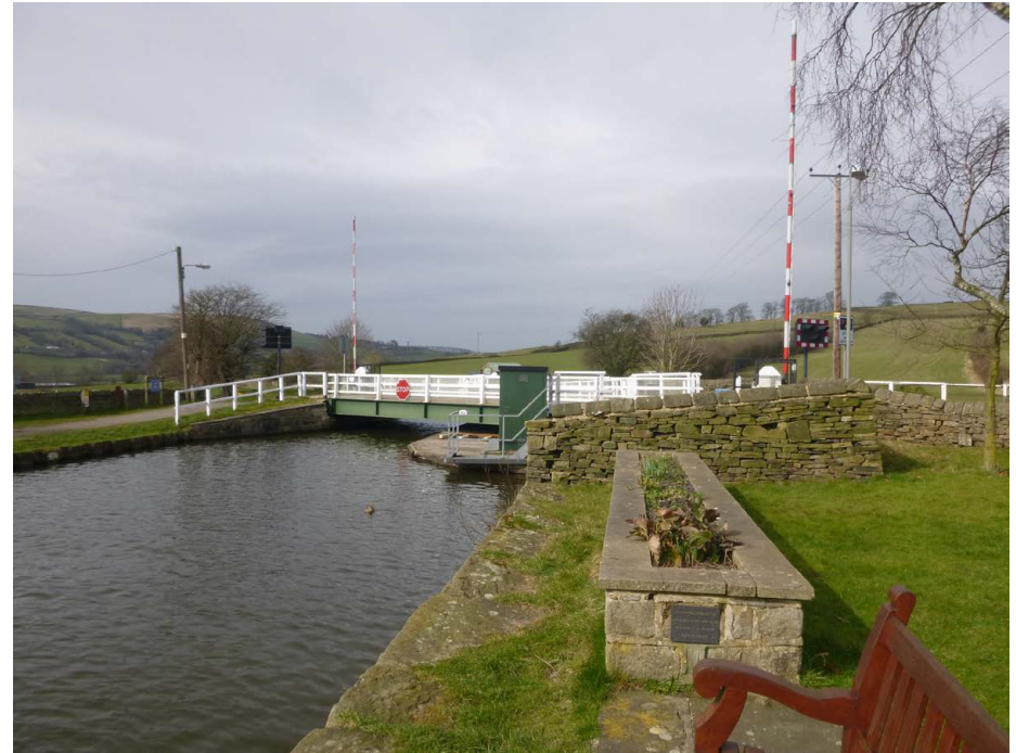
V13 along the Leeds Liverpool Canal with the Ings Lane swing bridge in the foreground
