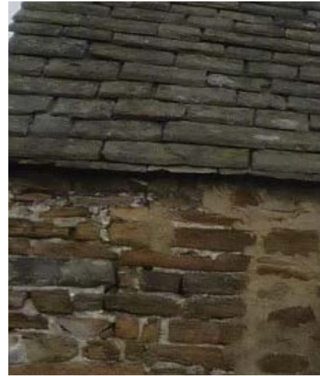
Grey stone slates (Yoredale sandstone) on a building in Low Bradley
