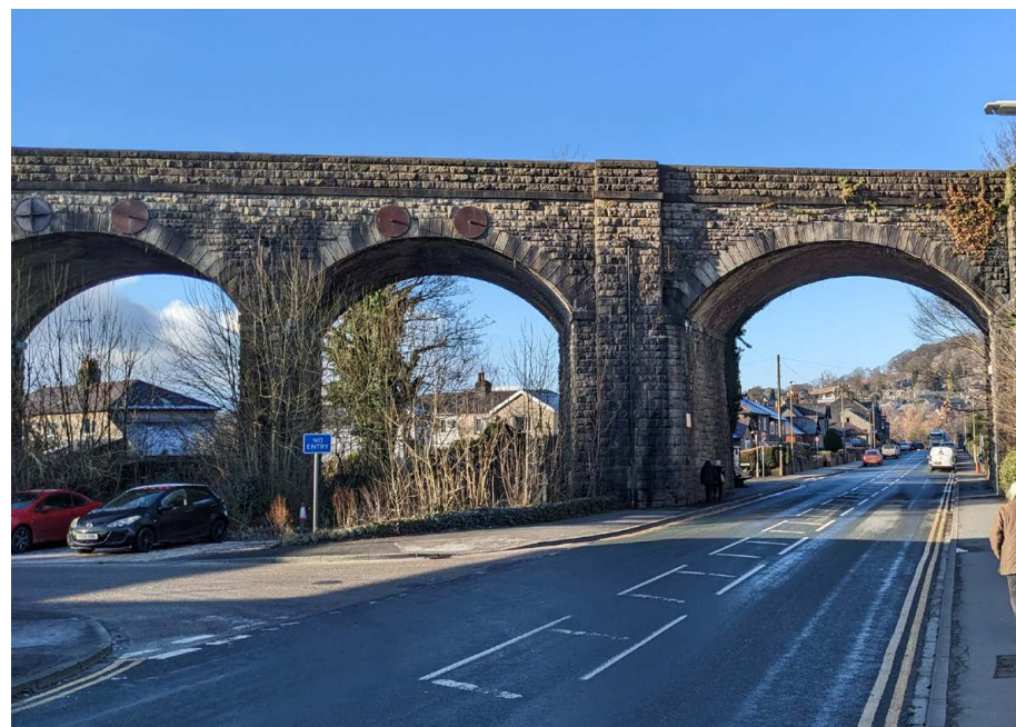
Church Viaduct, Settle (SAC/9) is the largest historic railway structure in the part of the Conservation Area that is in Craven
