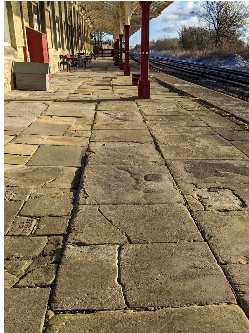
Hellifield Station retains its original sandstone platform paving, a rare survival
