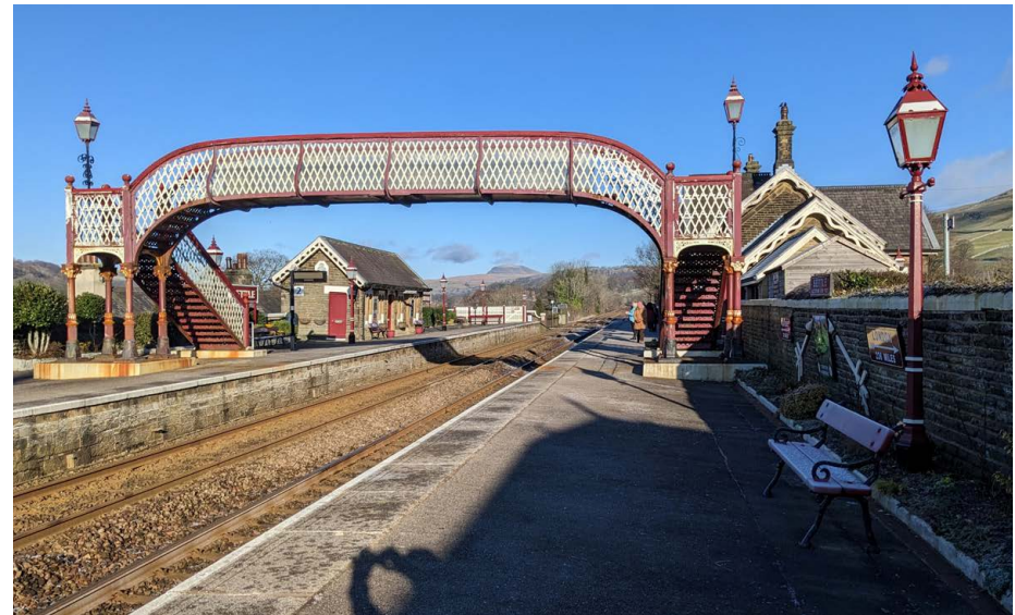
Settle Station is one of the best preserved historic stations on the national railway network
