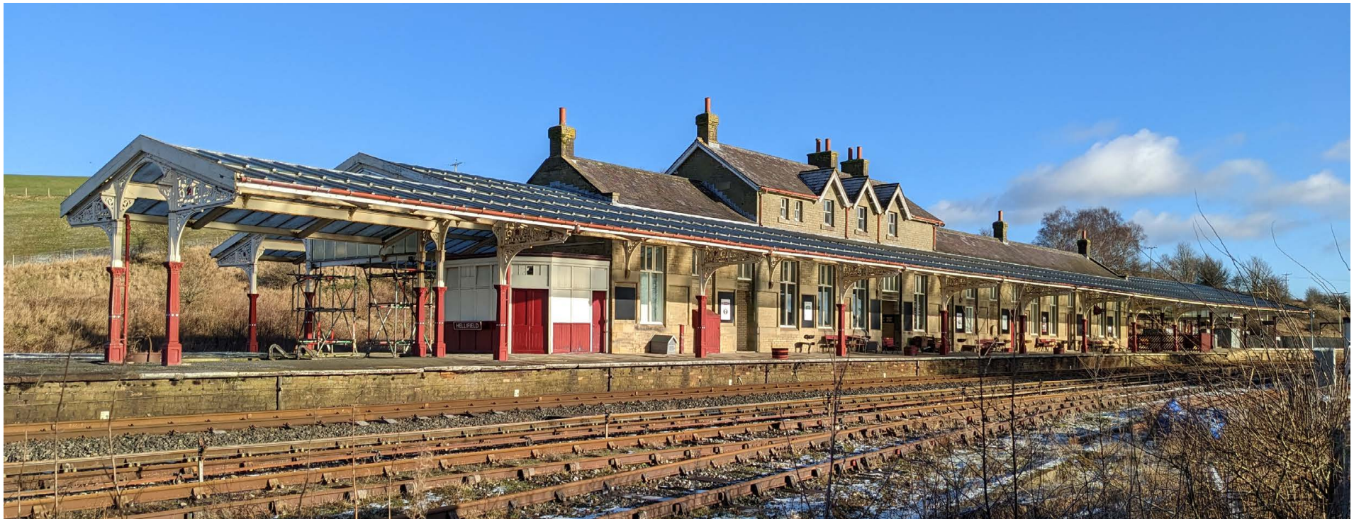
Hellifield Station has extensive iron and glass canopies
