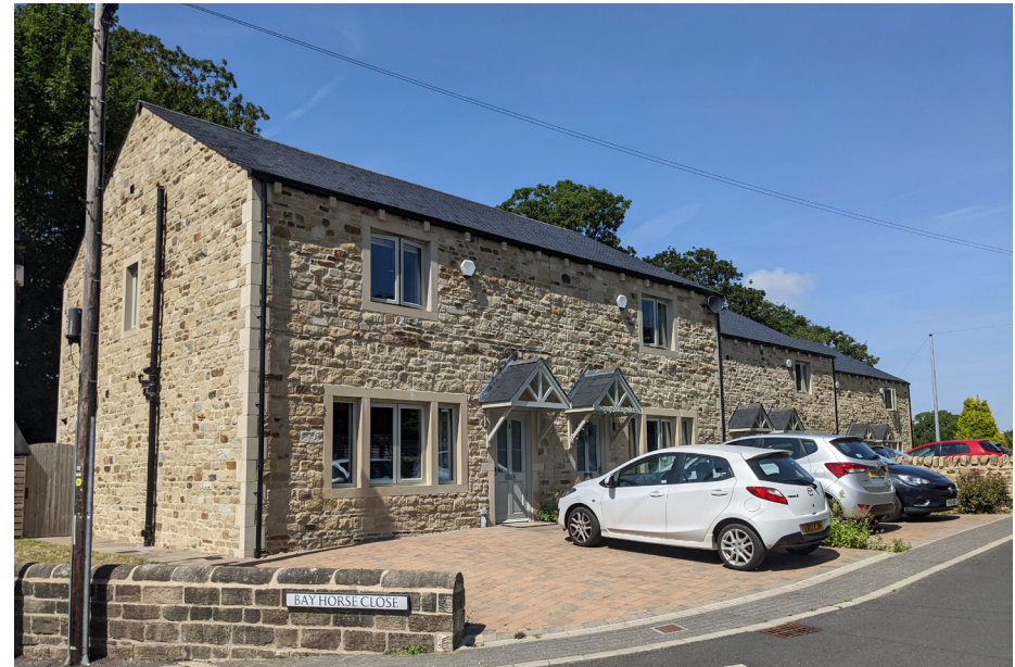
New build terrace (since 2016) on the site of the former Bay Horse Inn car park. Note the blue slate, timber porches and upvc windows and doors
