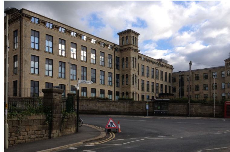
V6 - A strong view of the converted Greenroyd Mill from the junction of Holme lane and High Street
