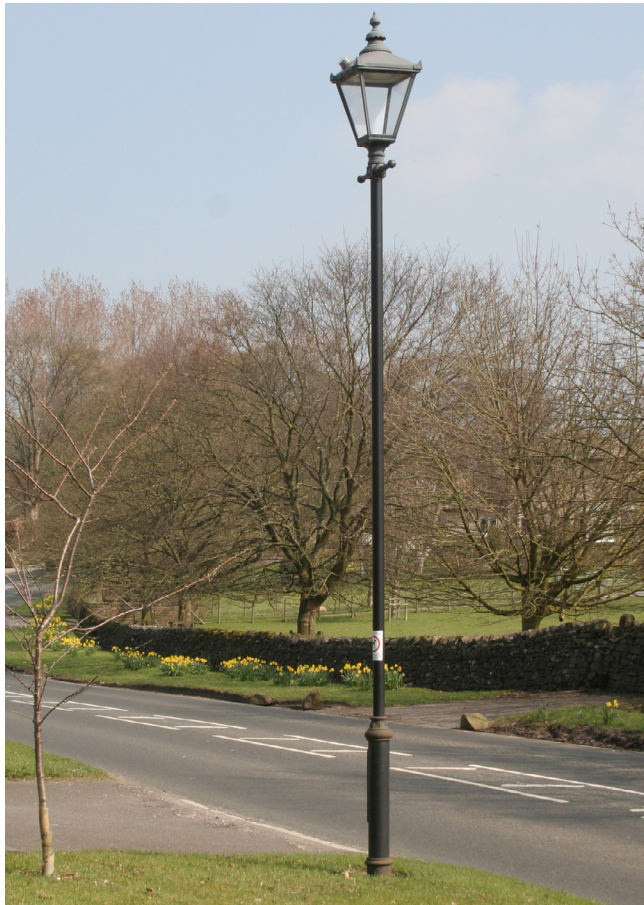
An example of a 'heritage' style lamp post
