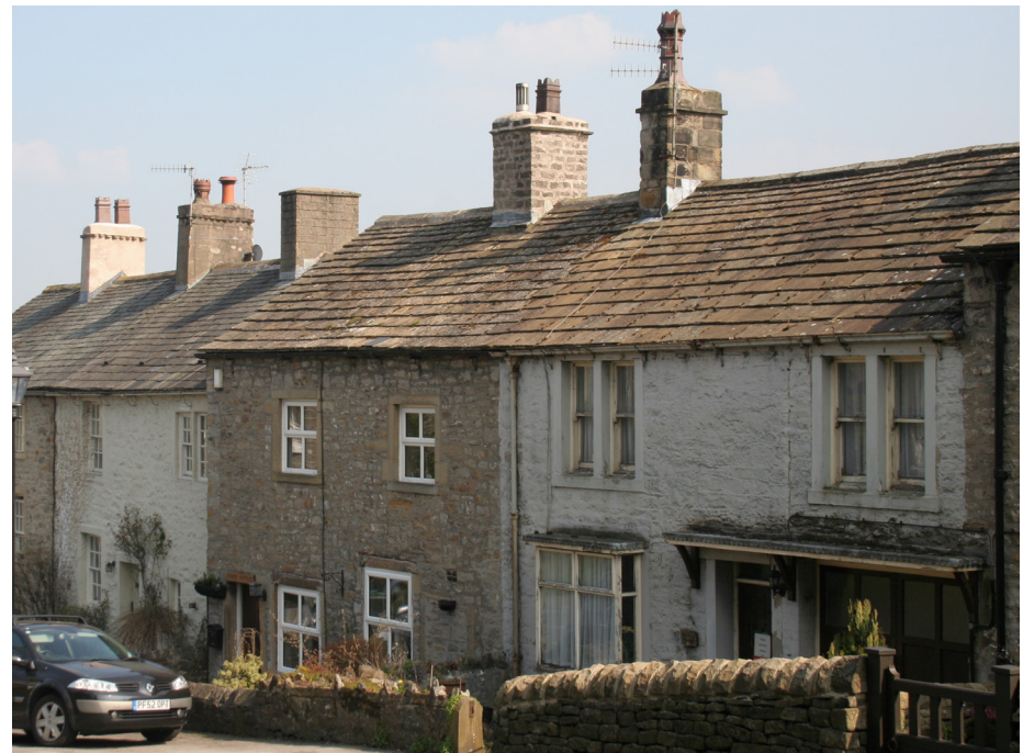
Traditional timber sashes and replacement upvc windows visible in this photograph. Note the stone slate roofs
