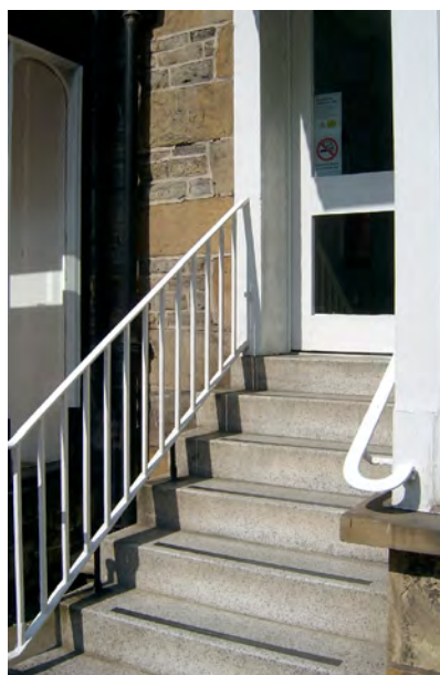
80. inappropriate material for steps, Middle Row
