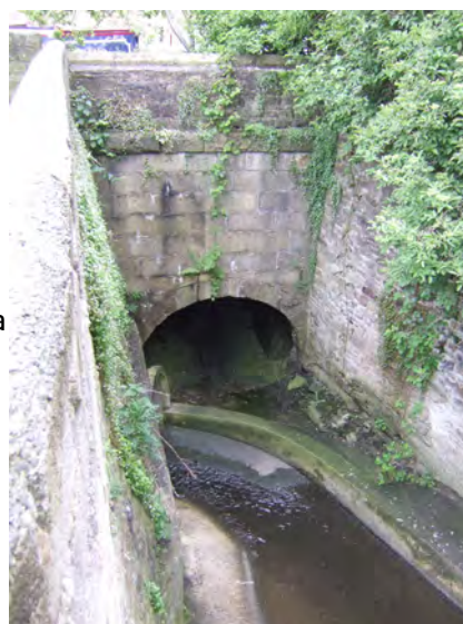
52. Waller Beck is culverted under the canal aqueduct and car park beyond
