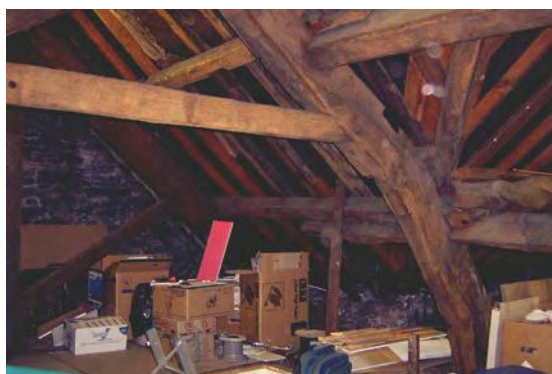
81. Cruck truss at the Cock and Bottle
