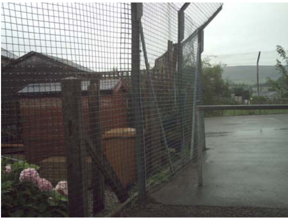
Figure 17. The location of the site is very close to houses which may be the reason for complaints to the police in the past.
