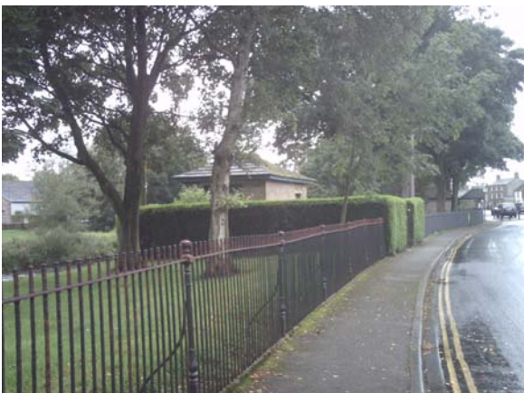
Figure 29. This is an image of the substation that residents are said to want demolishing, it is hidden behind fences and shrubs.
