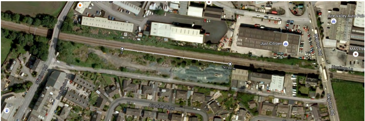
Figure 3 - Photo to indicate the platform length potential between structures
