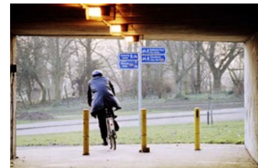
Bollards should be used to prevent vehicular access - York University. Note the removable unit for vehicle access
