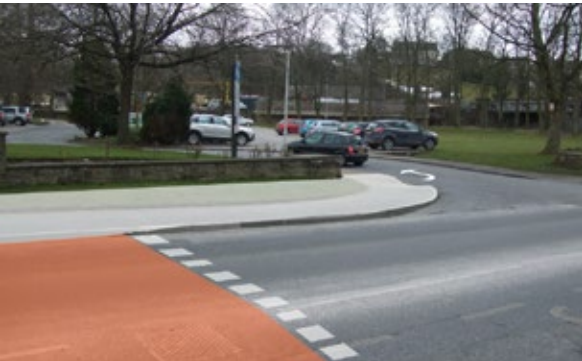
Link through hospital car park, create shared use link path on far side green verge to dropped kerb crossing point
