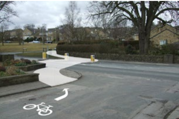
Create dropped kerb waiting area for cyclists, lengthen central reservation to the right to give easier cyclist crossing, convert far footway to shared use then reintroduce cyclists to Rockwood Drive carriageway
