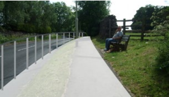
Widen the footway into verges both sides and retain against carriageway and guardrail. Move light columns and bench back
