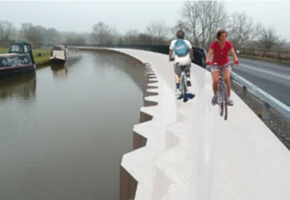
Remove railings, slightly narrow canal and widen towpath by creating new sheet piled wave wall further into canal to achieve min 3m wide space for towpath.
