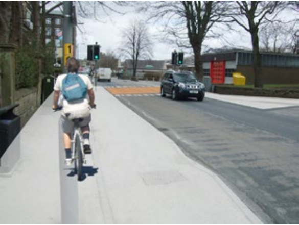
Access to station - Convert footway to shared use, relocate lamp column, convert pedestrian crossing to toucan, widen footway on far side to give better access to station car park from crossing.
