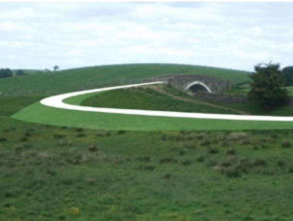
Create new better graded ramp joining bridge to towpath by acquiring a small area of adjacent field slope.
