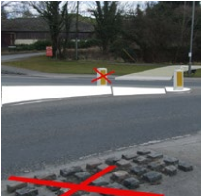
Realign crossing by removing 3m length of raised setts nearside, extend and widen central reservation, widen dropped kerbs both sides, create new path link from towpath to crossing on far side
