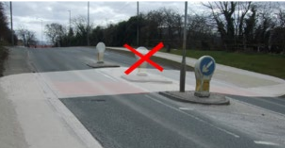
Widen canalside footway (on left) to min 2.5m, lengthen central reservation, improve footway splay on far side
