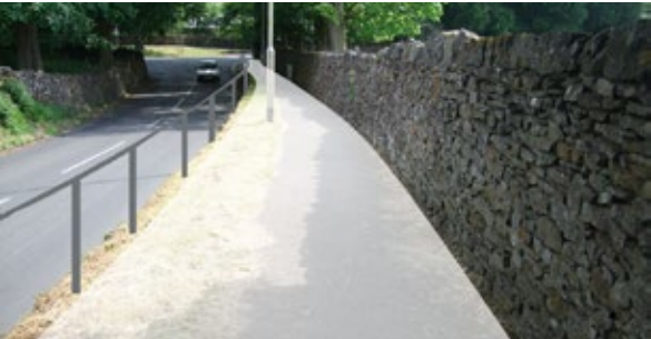
This footway could be widened using the grass verge and moving light columns to the back of the footway. A guardrail could be installed where necessary.
