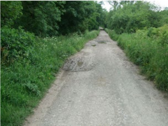
Bank Newton Lane example of pot-holes that would require repair.
