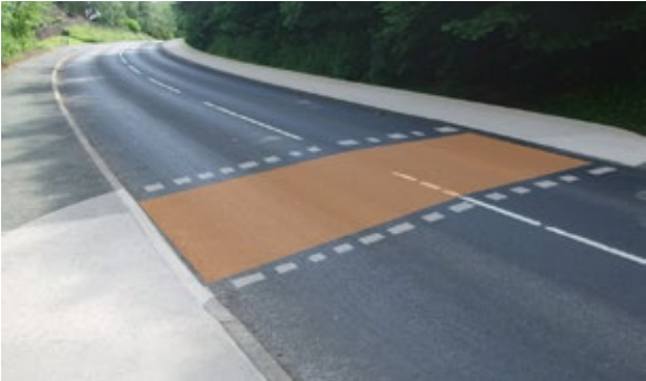
The shared use footway would cross using widened dropped kerbs.
