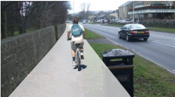
New Central reservation crossing of Keighley Road, convert footway to shared use, widen where necessary to 2.5m min
