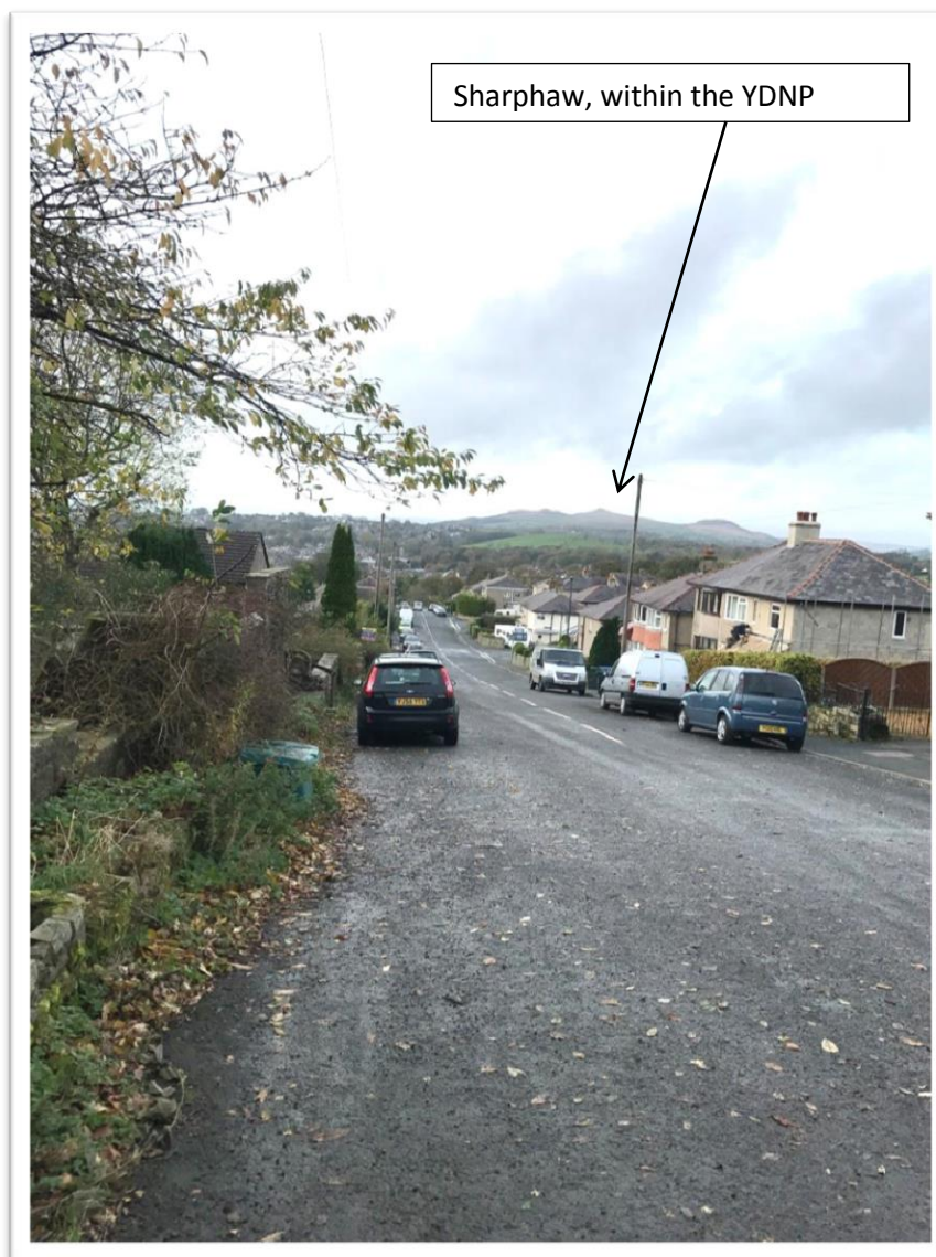
Fig 7.3 long distance view of Sharphaw in the YDNP from the northern site boundary of site SK015
