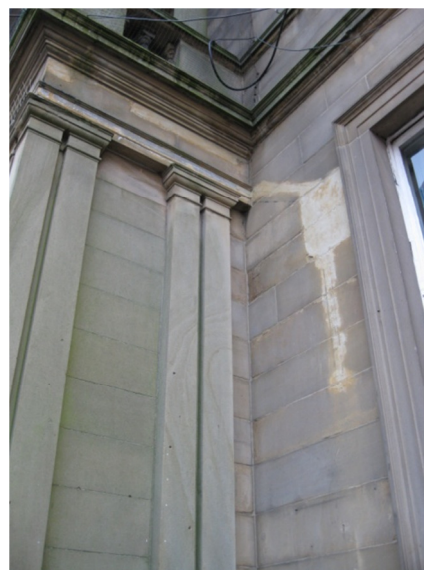
Fig. 34 Front wall: loose wires, redundant fixings, and poor repair following removal of the glazed canopy in 1956.
