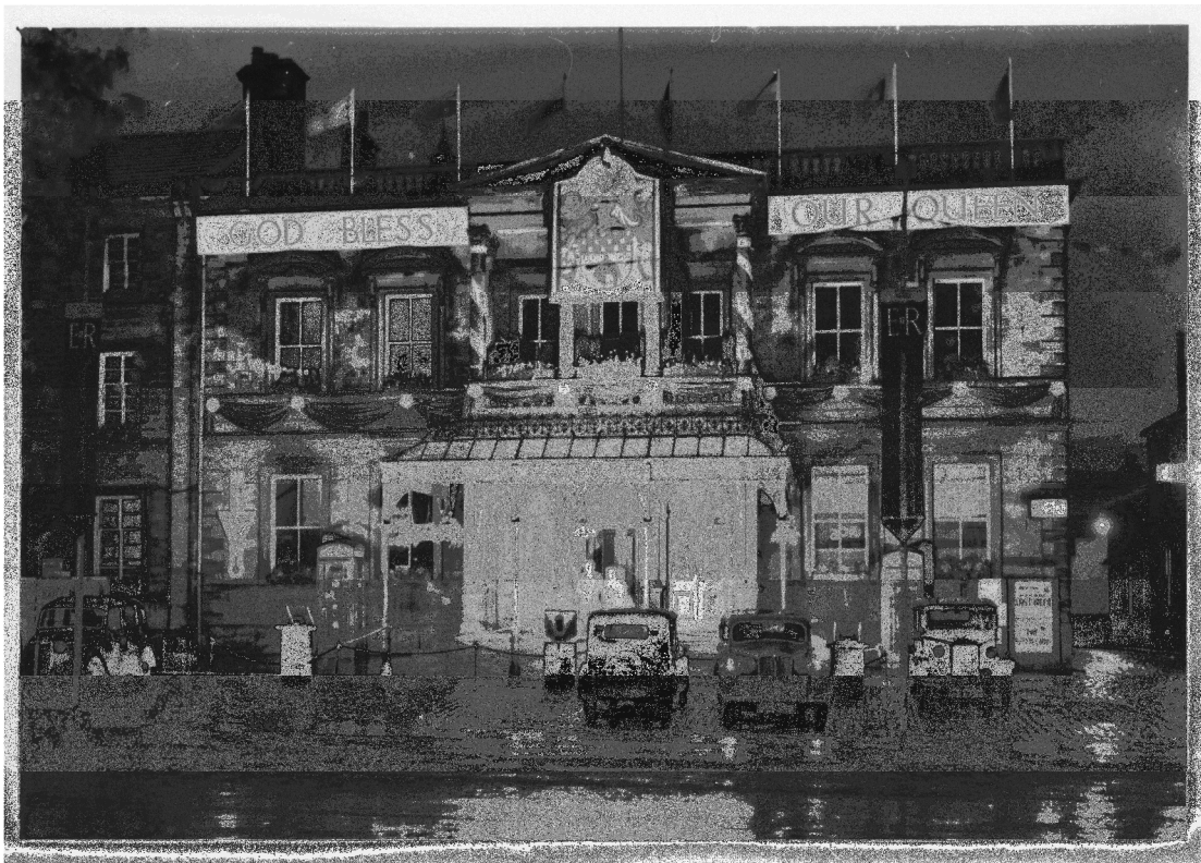
Fig 21 Archive photograph showing the decorated front in 1953. The canopy gas-lights have gone and structure was removed in 1956 after repeated damage by cars.
