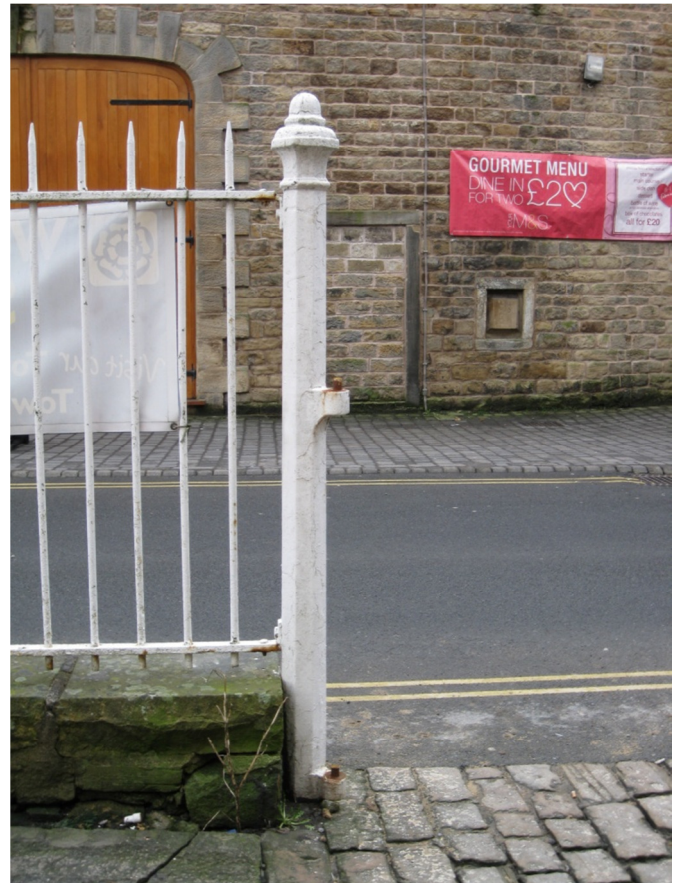
Fig 7 Original gate post south side, probably re-positioned c1960.
