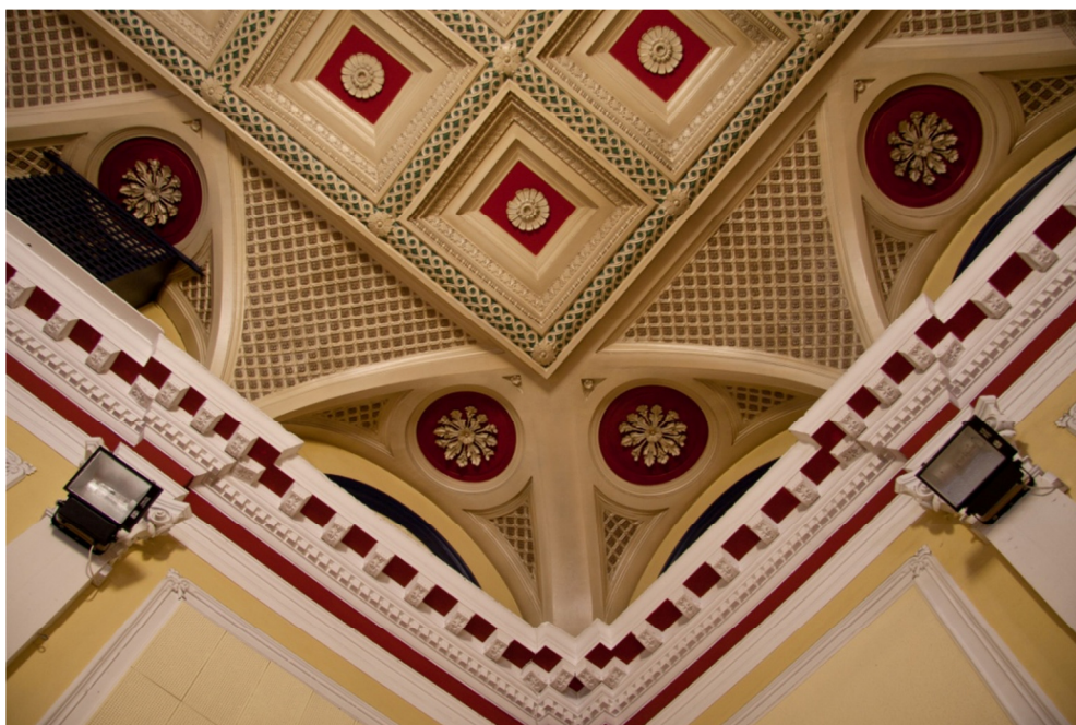
Fig. 34 Main hall ceiling detail. See Appendix 1, Room G23. High Victorian decorative plasterwork, 20 th century colour schemes.
