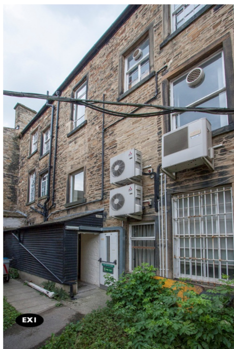
Fig. 32 Rear view of the Big Entry. 20 th century needs for access, ventilation and security have almost destroyed the attractive balanced elevation. Compare with Fig.9.
