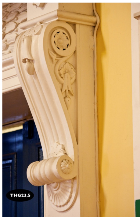
Fig 19. One of the elaborate console brackets for the main concert hall entrance. A list of the craftsmen working on Lockwood & Mawson’s new hall was published in the Craven Pioneer on May 8 th 1875. Joinery was by J.Pettyt of Skipton, Benjamin Dixon of Bradford did the plasterwork. RH
