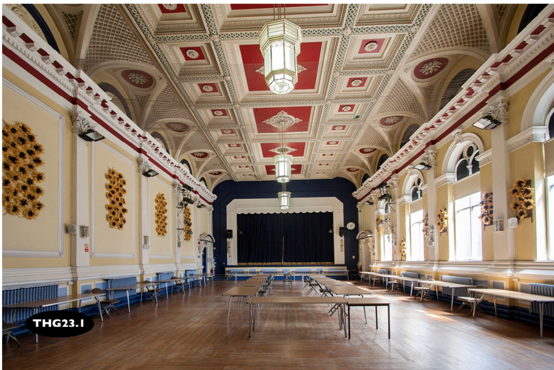
Fig 20. 1876 hall; lights and proscenium arch probably 1933, when the pillars were marbled and the stage made larger. Maplewood floor 1956. Poor later treatment with insensitive down-light fittings, blocked upper window lights, netting to catch falling plaster, mouldings cased in, colour scheme highlighting ugly radiators, inappropriate decorations. See Appendix 6 Time-Line and 11 archive photographs for the 1927 interior. RH
