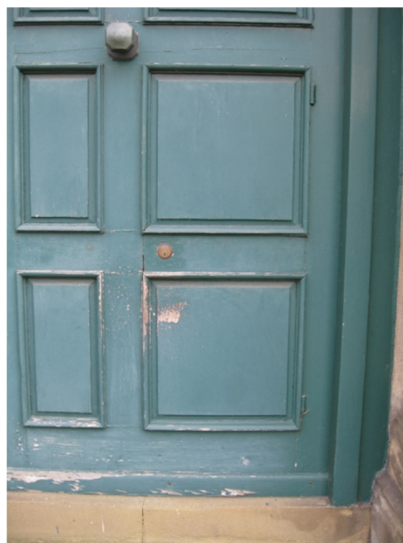
Fig. 8 Wicket-gate in double doors of the 1838 Big Entry. Doors sealed up in 1962 when the staircase was inserted into the passage and the building was linked to the 1862 Town Hall. The door style dates from the 1930s.
