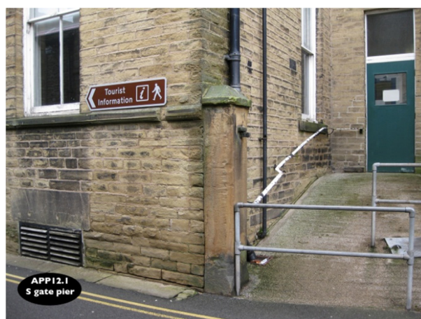
Fig. 33 Entrance from Jerry Croft. Blackened walling reveals the old boiler house cellar ventilation. An original stone gate post (see Fig.17) and ugly pipework, handrail, safety fence, emergency exit. Original area steps to the basement survive under the steep concrete ramp. See App 1 Rooms B4 and B5.
