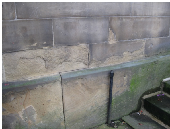
Fig. 33 Front wall base next to the entrance steps: surface stone erosion and lamination.
