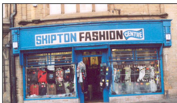
Skipton Fashion Centre – shop front in need of modernisation.
