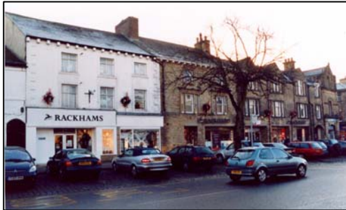
Rackhams Department Store
