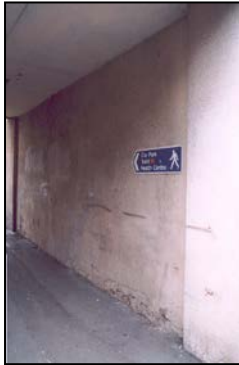
Main car park, access
