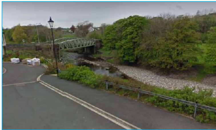
Figure 12 - New Bridge River Greta (©Google 2017)
