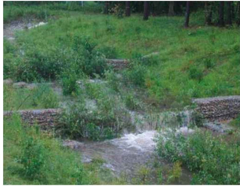
Stone weirs within the drainage channels
