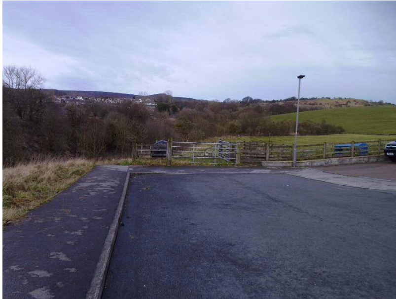
Figure 11: Existing Stub Road Carriageway on Airedale Avenue
