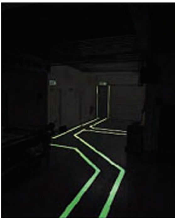
Figure 52: A 'way-guidance' system
