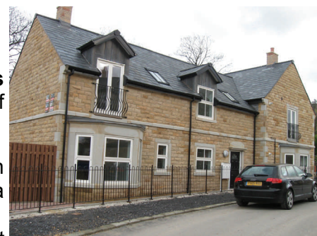
New house completed on brownfield land at Greenroyd Mill, Sutton
