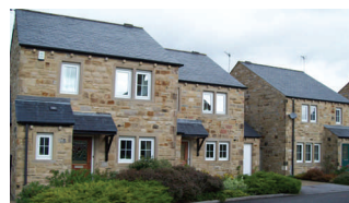
Affordable housing provided at Lord's Close, Giggleswick
