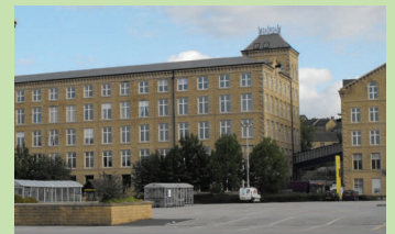
New housing completed at Belle Vue Mills, Skipton
